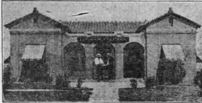
Local office at Flossmoor Park
